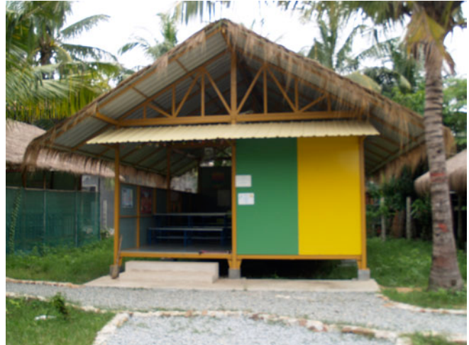
Classroom - electrical and wood turning workshops are completely enclosed for security reasons
